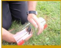
peg through thr ough the hole in both the Prepex and the conduit. Make sure the top of the peg sits
